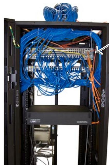
The horizontal cable management tray keeps cable from falling in front of other things in the rack.
